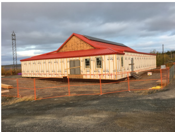
Museum construction August 2018
